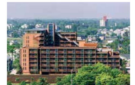
Ninomiya House International Residence for Researchers
