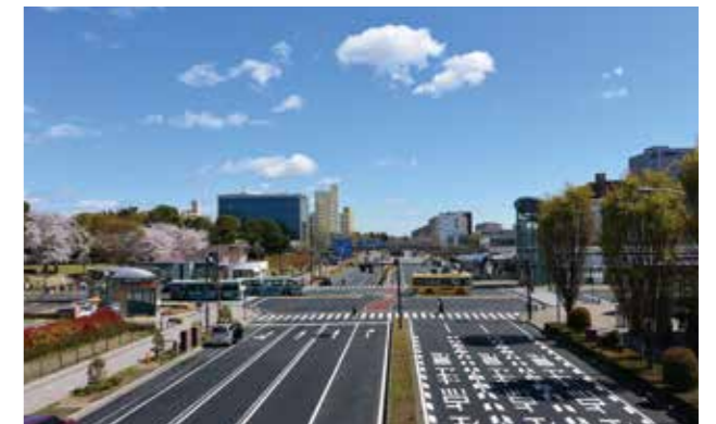
Front area of TX Tsukuba Station, where electrical cables have been relocated underground
